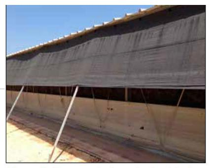
Figure 9. Porous window shades block direct sunlight from entering the house, ass through.
