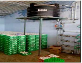
Figure 12. Having the water tank inside the house keeps the water cooler.
