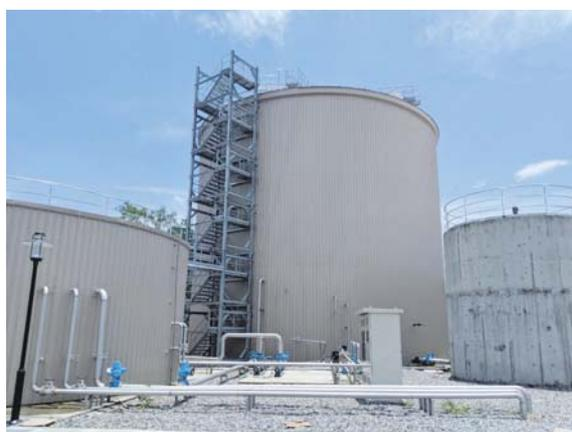
*Anaerobic co-digestion tank in Tai-Sugar Company*
