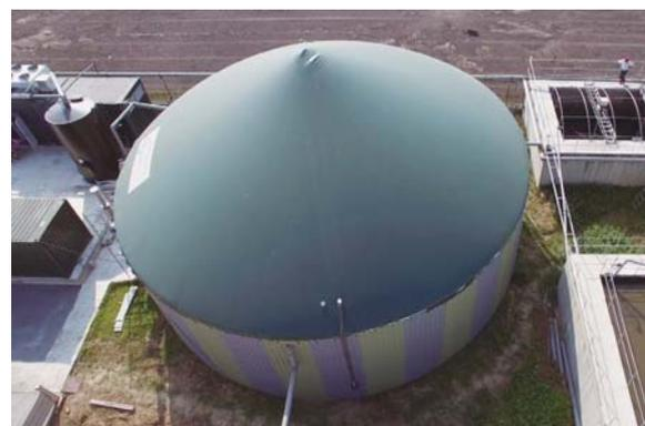
The continuous stirred tank reactor
