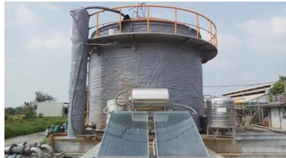
*The continuous stirred tank reactor and preheating facilities*
