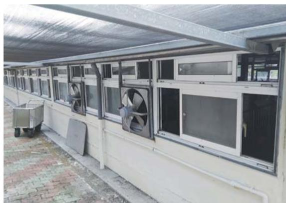
*Intelligent temperature monitoring and control fan system set in the nursery pig house*
