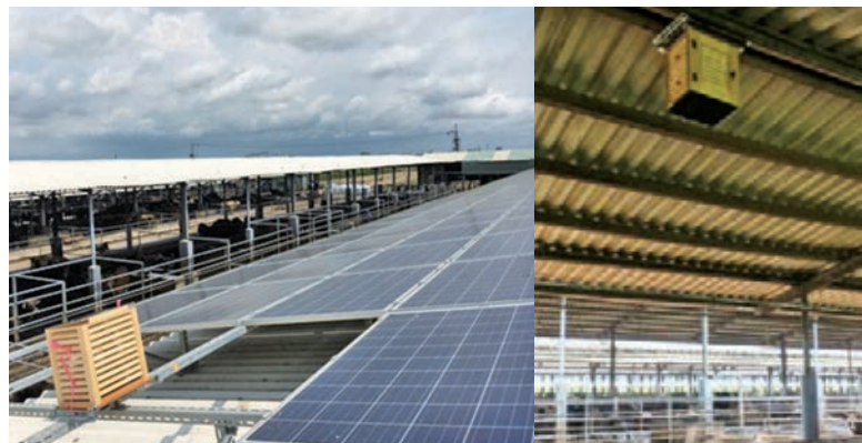
Louvered enclosures housing temperature and humidity sensors installed above (left image) and below (right image) the solar panel roof
