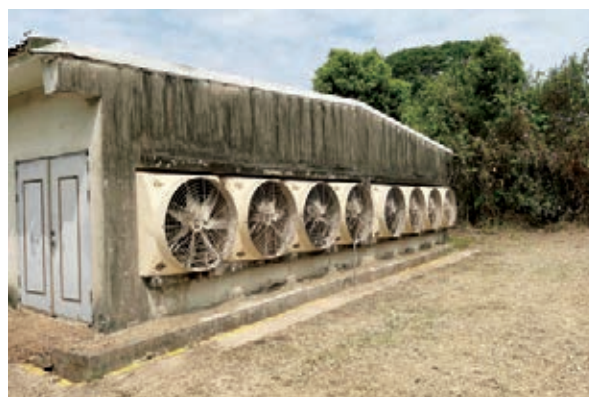
The variable frequency exhaust fans after improvement in laying hen houses
