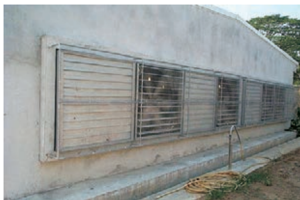
The original constant frequency exhaust fans before the improvement of the laying hen house
