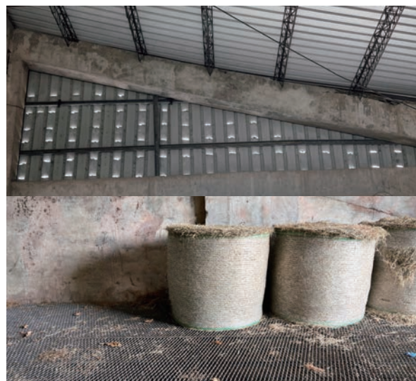
The corrugated steel sheet under the roof (up) and the floor below were provided with holes (down) to facilitate ventilation
